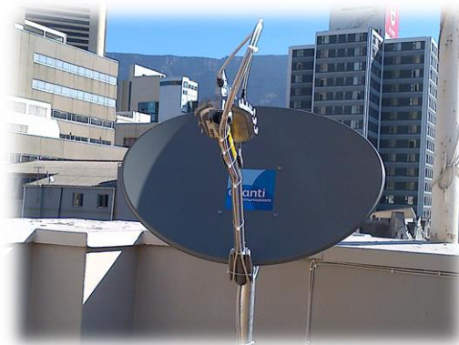
Data Network Environmental Services Cape Town South Africa
